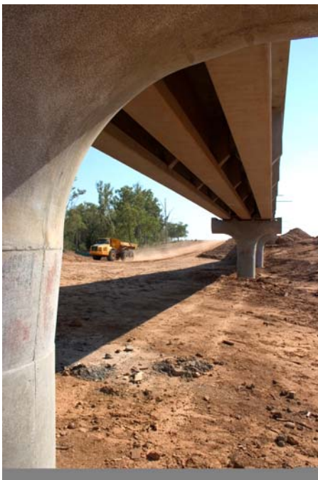
View from beneath the girders on a rail bridge
