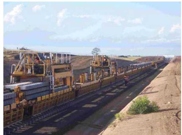
Above and below: Track laying machine in operation at the northern end near Kinrola.
