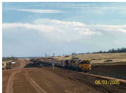
Sleeper delivery train at the back of the track laying machine
