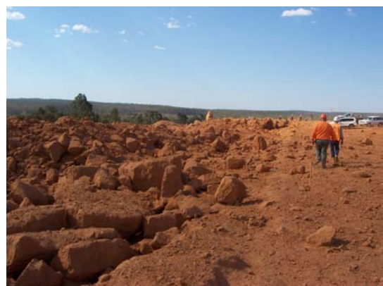
Earthworks cutting through the Central Queensland landscape
