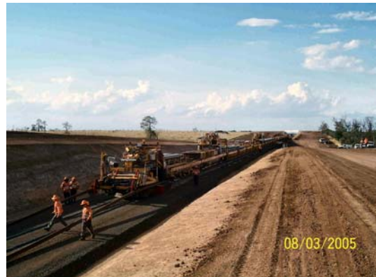
Above and below: Track laying machine in operation at the northern end near Kinrola.
