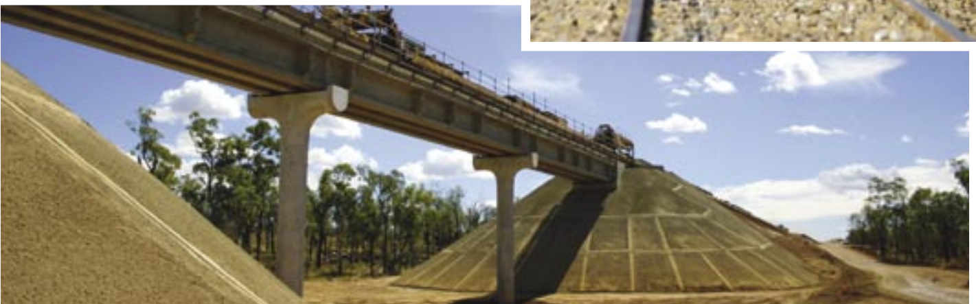
Track laying machine working across Horseplain Creek Bridge
