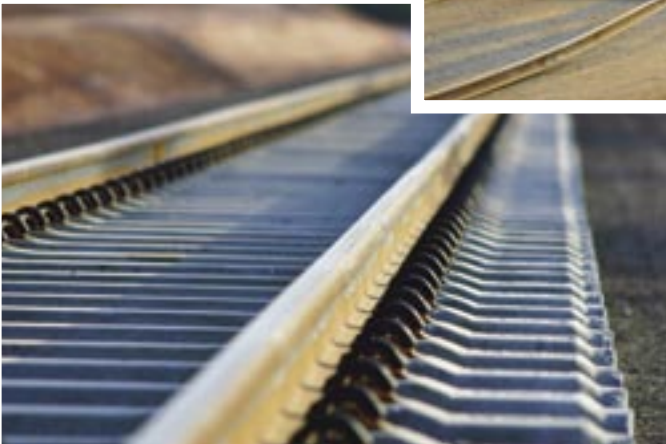
Early track laying before ballast...
