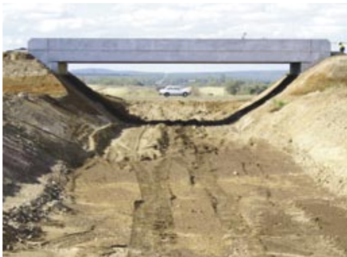
Dawson Highway Bridge, view from the south.
