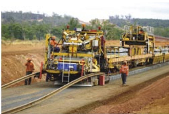
Track laying machine in action
