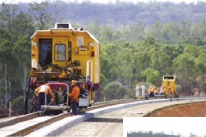
Flashbutt welding near Horseplain Creek Bridge
