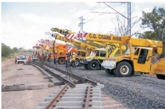
Duplication works at Tryphinia on the Blackwater Line
