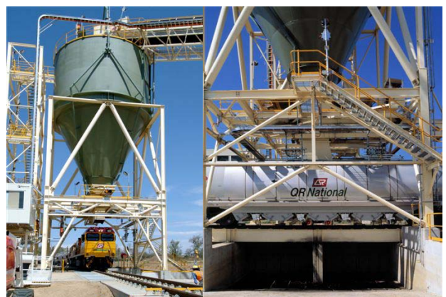
Loading coal onto the first train to depart from Rolleston mine.
